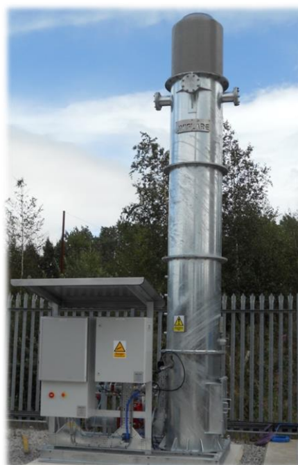
VAB installed near Doncaster, UK
